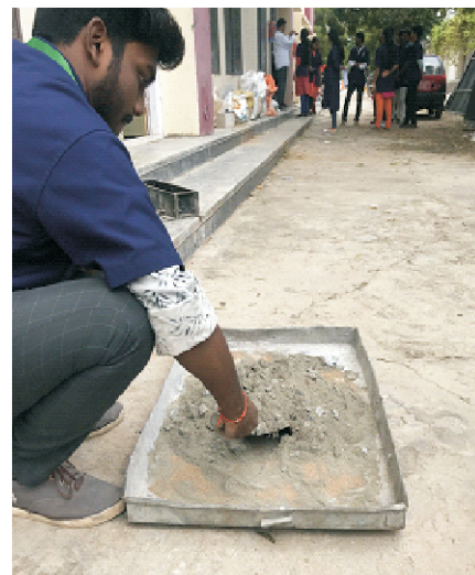
Figure 5. Mixing of Concrete
