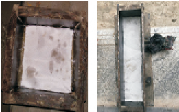
Figure 6. Placing of Geotextile in the Concrete Cube and Beam Mould
