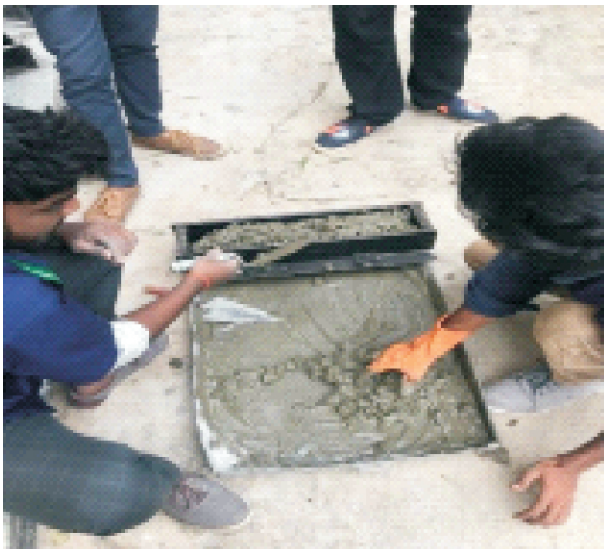
Figure 7. Placing of Concrete in the Beam Mould
