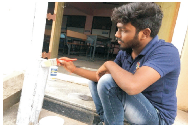
Figure 2. Application of Membrane Curing for Concrete
